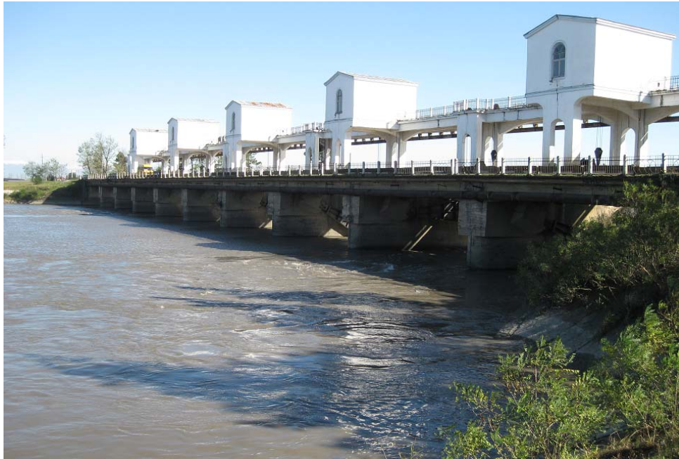
Fig. 5. The Downstream Wall of the Rioni Water Dividing Structure
