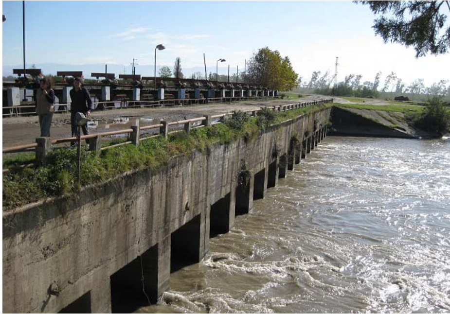
Fig. 6. Headworks of City Canal
