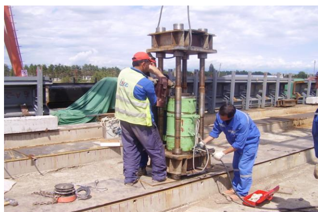
Photo 1. Steel frame for calibration together with YDT 3000 jack
